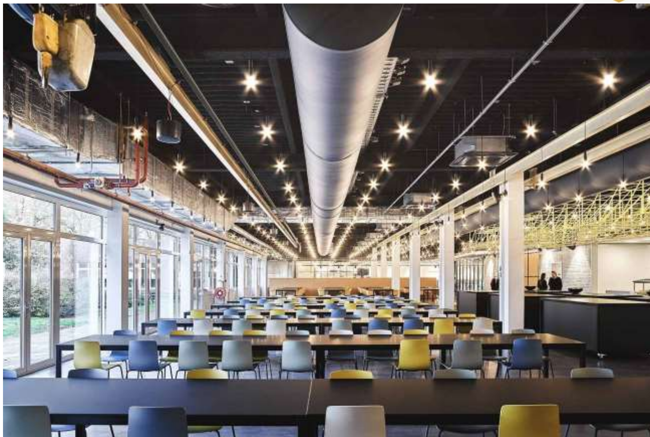
PROSPRAY in black to corrugated metal ceiling.
