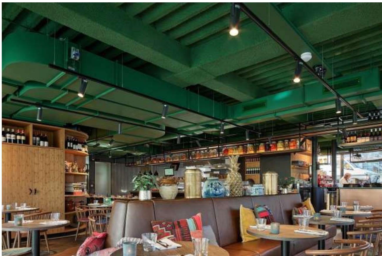
Proplaster in bespoke colour directly applied to uneven surface
